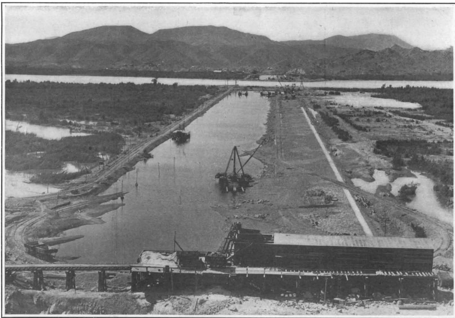
Dam partly completed. Note top of core wall, and, in right foreground, the stone paving.
