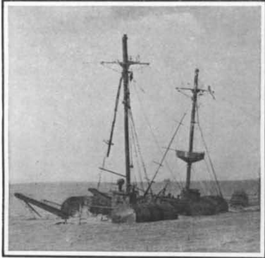
The "Gladiator" righted. The derrick, now nearly horizontal, may be seen on the left, and the "camels" on either side.
