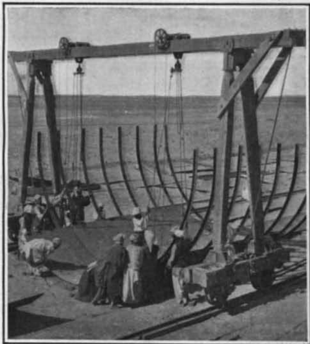
Affixing Plates to the Ribs.
