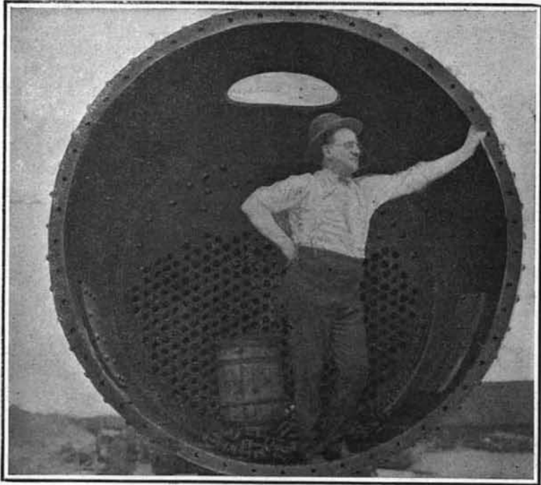
View Looking Into Smokebox, Whose Diameter is 8 Feet.
