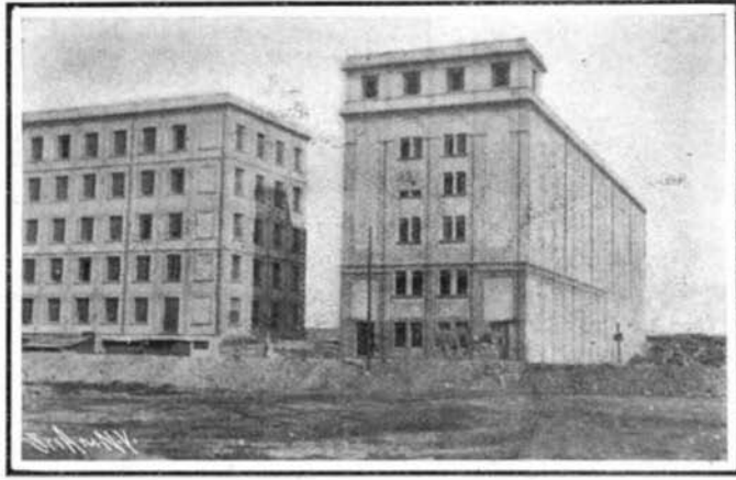
The Structure After Being Raised to Its Normal Position.
