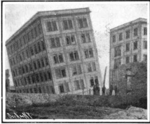
Extreme Displacement from the Vertical.
