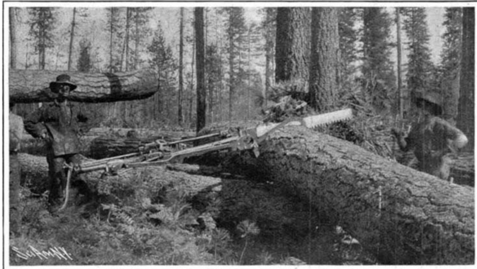
The Compressed-Air Logging Saw in Operation.
