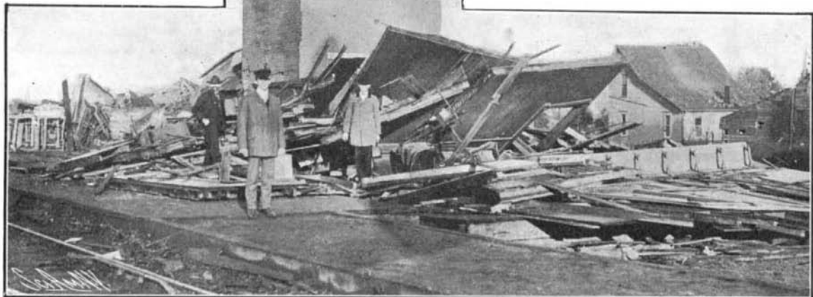
Scene at the Railway Station, Showing the Ruins of the Depot and What is Left of the Grain Elevator.
