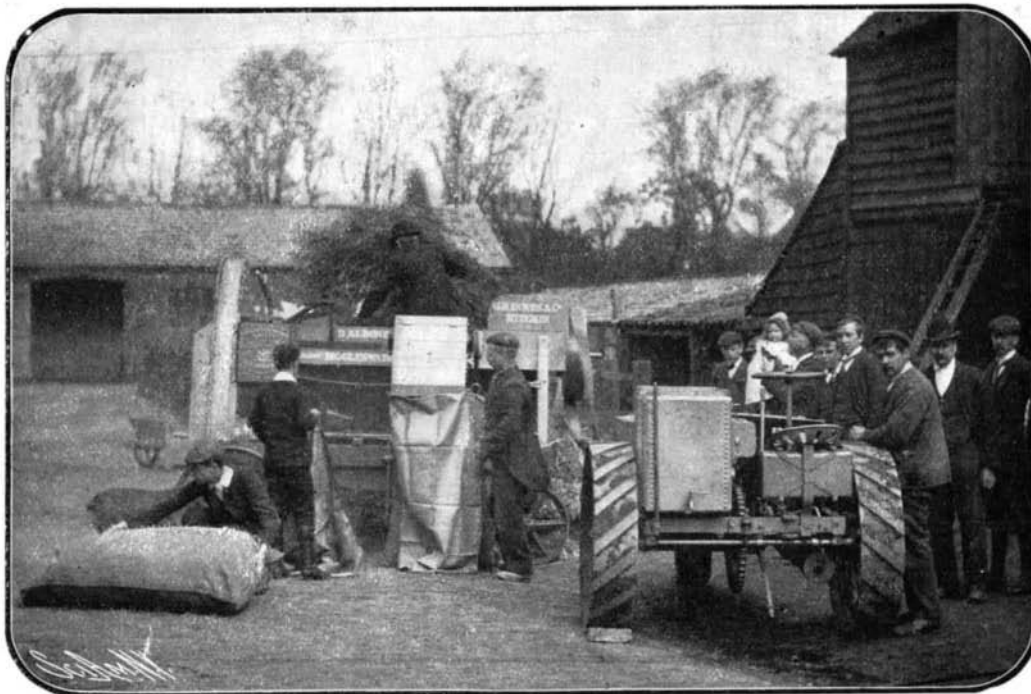
THE IVEL MOTOR DRIVING A THRESHING MACHINE.
