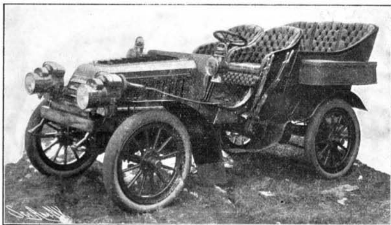
THE MITCHELL AIR-COOLED FOUR-CYLINDER TONNEAU.
