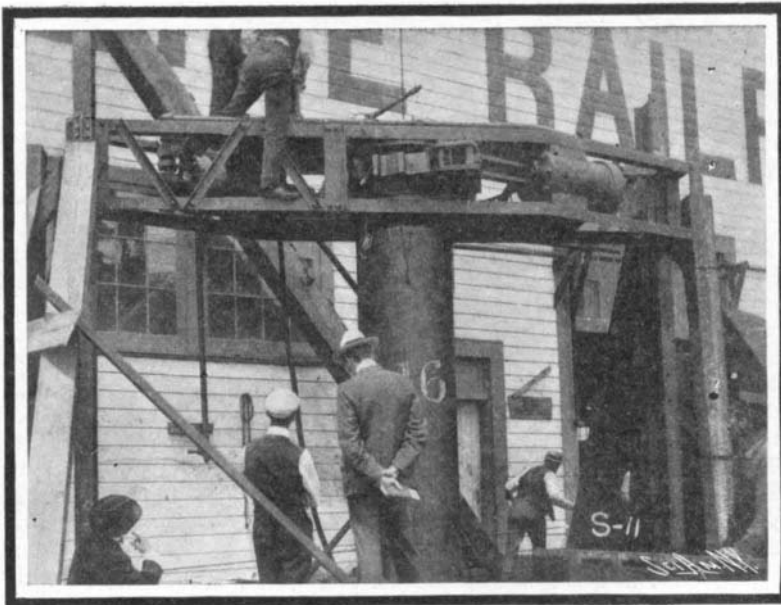
View of Top of Pile, Showing the Hydraulic Screwing Machine.
