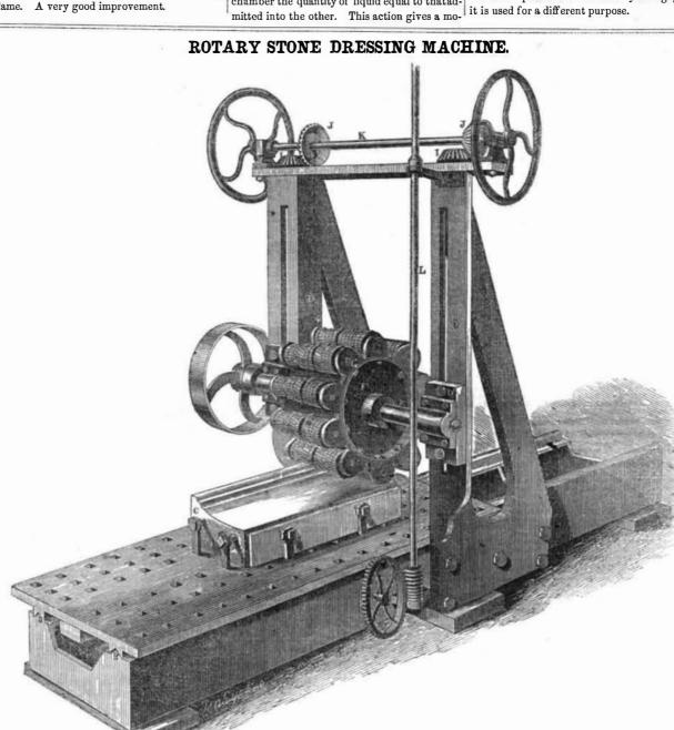
grooved or burred faces, made of cast iron and with bevel pinions, J J, meshing into others, I chilled, are strung, as it were, on a series of I, on vertical spindles, which have screws spindles, around a drum; the drum is revolved, upon them working into nuts, (not shown,) and are a composite of iron and steel.
