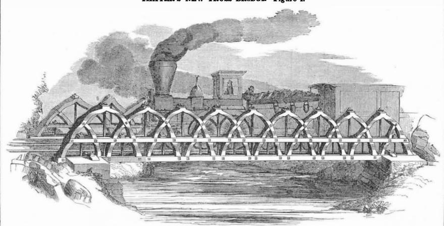
The annexed engravings are views of an improvement in the truss for iron bridges, roofs, &c., for which a patent was granted to G. W. Thayer, formerly of Springfield, but now of Hartford, Conn., on the 11th of last April,
