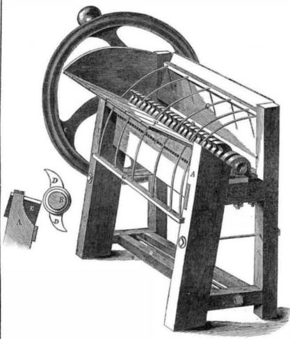
spective view of a Straw and Vegetable Cut- presses it and carries it downward to the feed ter, patented Dec. 21st, 1852, by W. Gale, of ing hooks. Louisville, Ky., now residing in Troy, N. Y. The knives are so constructed that when The machine is of a novel construction and its broken, the ends may be readily changed or operation is efficient.
