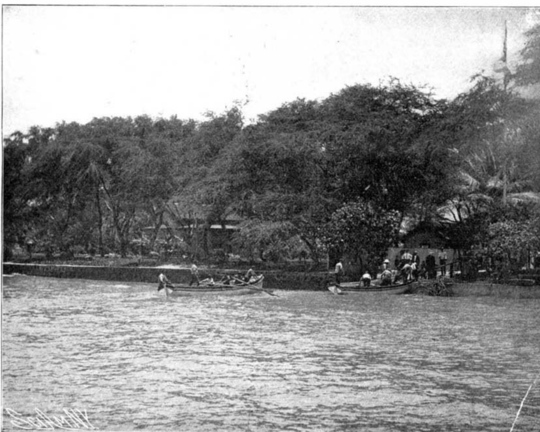
Boats Landing the Light Line, by which the Heavy Hawser to which the Cable is Attached is Hauled In.
