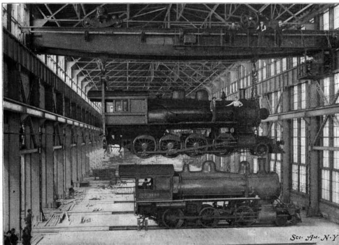
LIFTING AN EIGHTY-TON LOCOMOTIVE WITH A TRAVELING CRANE.
