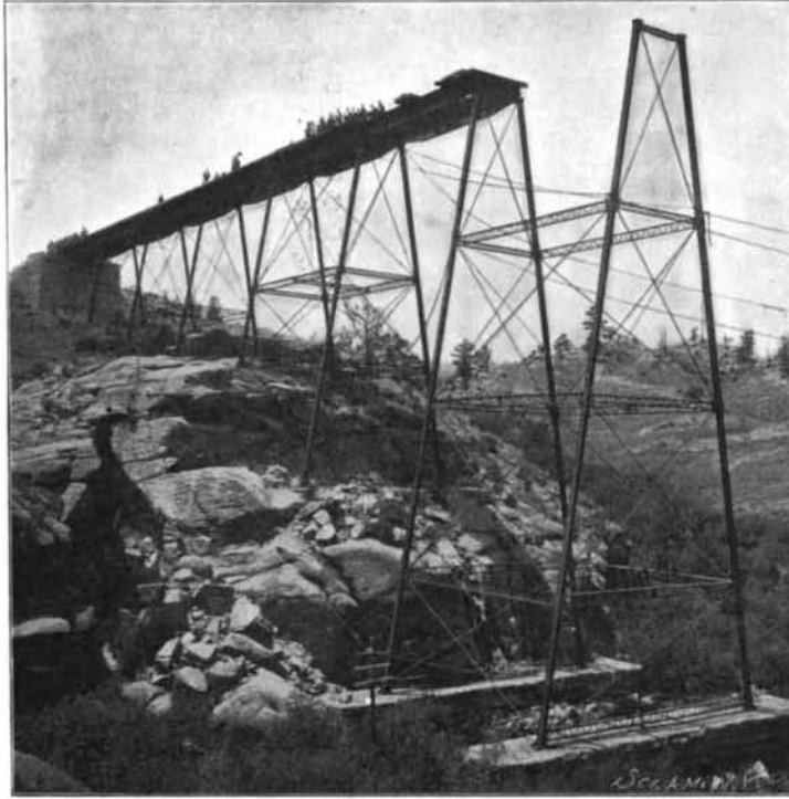
Removing the Old Dale Creek Bridge.
