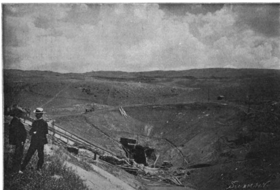
Photographs by J. E. Stimson. West Entrance to the Aspen Tunnel.
