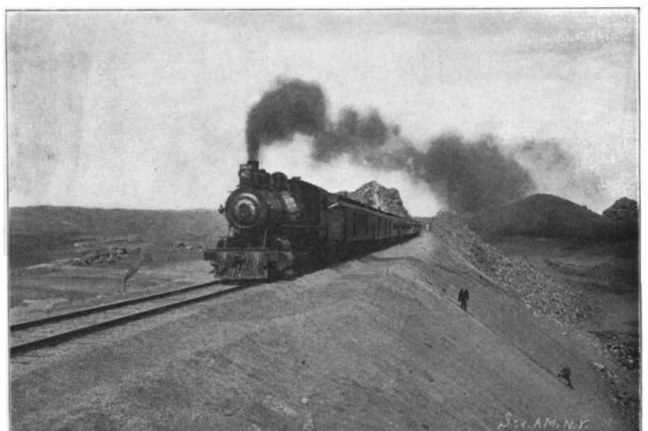
Dale Creek Fill; Buford-Laramie Cutoff. Height of Fill, 120 Feet; Amount of Material, 500,000 Cubic Yards.
