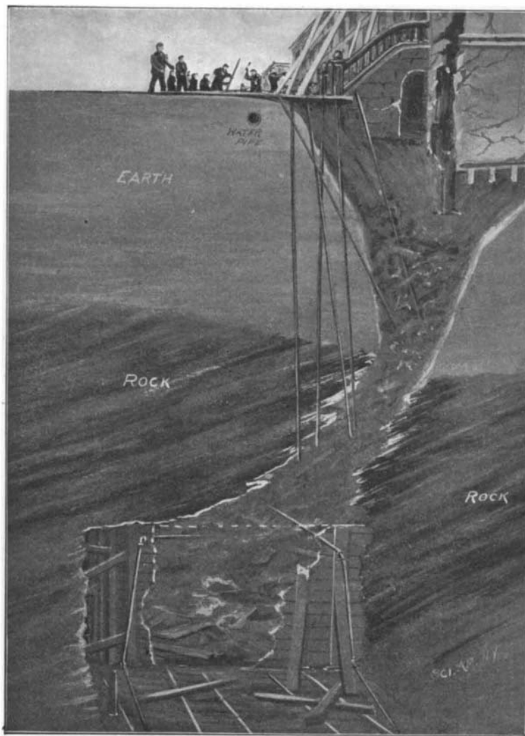
CAVE-IN, SHOWING THE METHOD OF REPAIRS BY BULKHEADING AND GROUTING.
