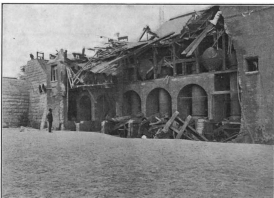
Wheelpits Exposed by the Fall of the West Wall of the Power House.
