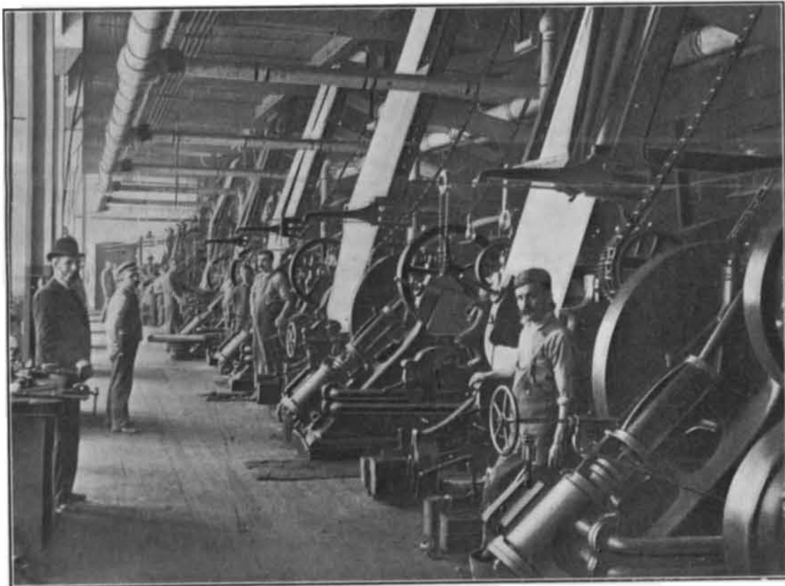
Cotton-Mill Printing-Machines Driven by Compressed Air Engines.
