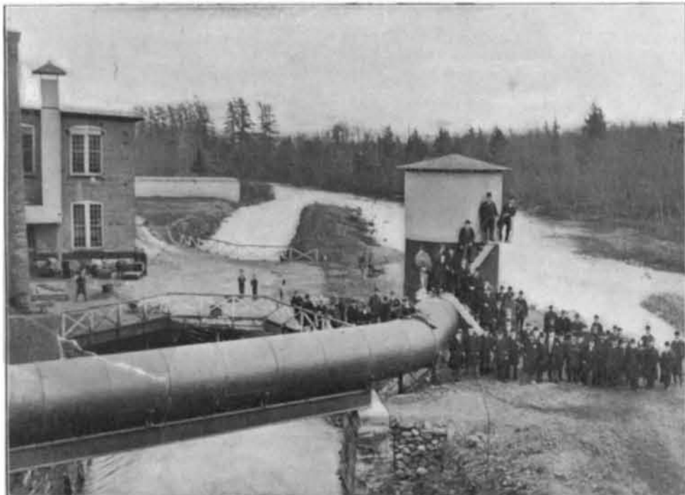
The Penstock and Receiving Tank.
