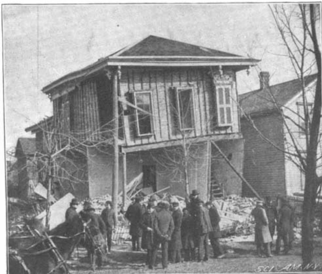
FRONT OF HOUSE WRECKED BY GAS EXPLOSION.
