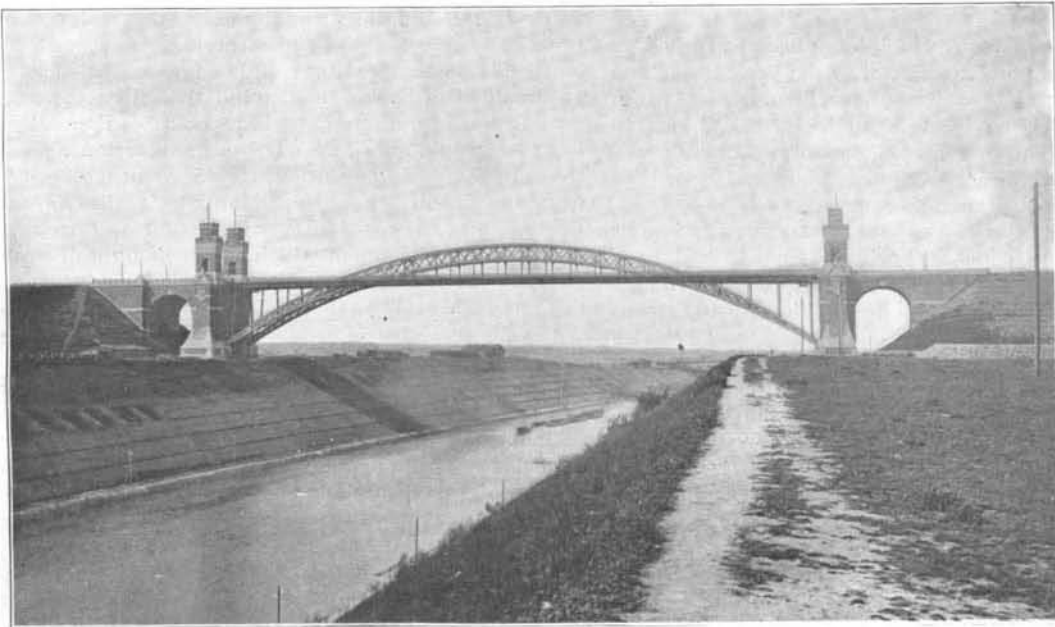
Grunenthal Bridge Across the Kiel Canal. Span, 511.7 Feet.
