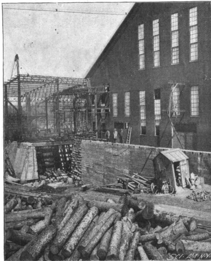
GATE HOUSE AND CONNECTING CANAL.
