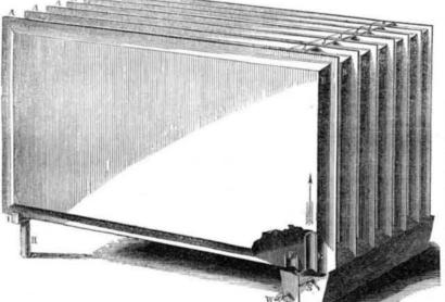
tive view, with a small portion of the shell removed, of the apparatus of Mr. A. S. Lyman, of this city, for heating apartments by steam, and for an exterior condenser tor steam engines.
