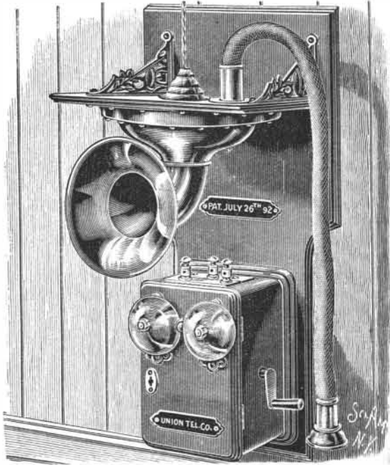
Fig. 2.—THE SIMPSON ACOUSTIC TELEPHONE—HORIZONTAL ARRANGEMENT.
