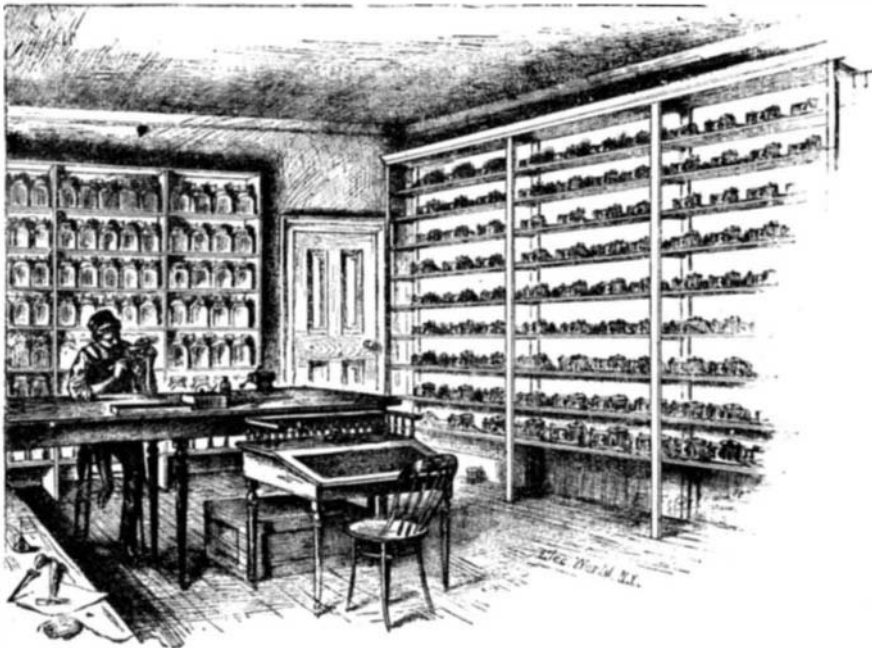
Fig. 3.—TELEPHONE CENTRAL OFFICE.
