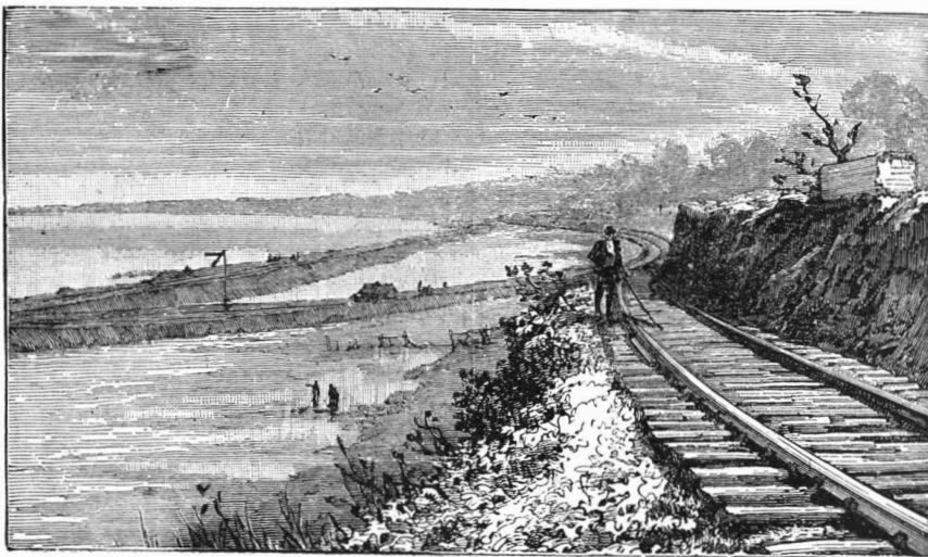
THE MERSEY ESTUARY WORKS NEAR EASTHAM.
