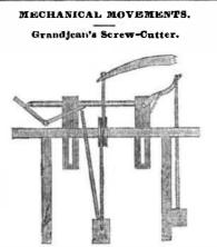
This is a machine which was proposed and used in France during the last century, invented by a gentleman named M Grandjean, for cutting screws. The piece of iron to be cut was traversed by means of the bent lever on the left which was acted on by the treadle which gives the rotary motion by the cord round the pulley. Those who would cut the head off all improvements as infringements upon old principles, have just to compare the above with modern machinery for cutting screws.
