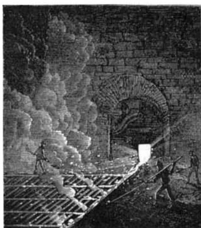
FIG. 5.—RUNNING METAL INTO PIGS.
