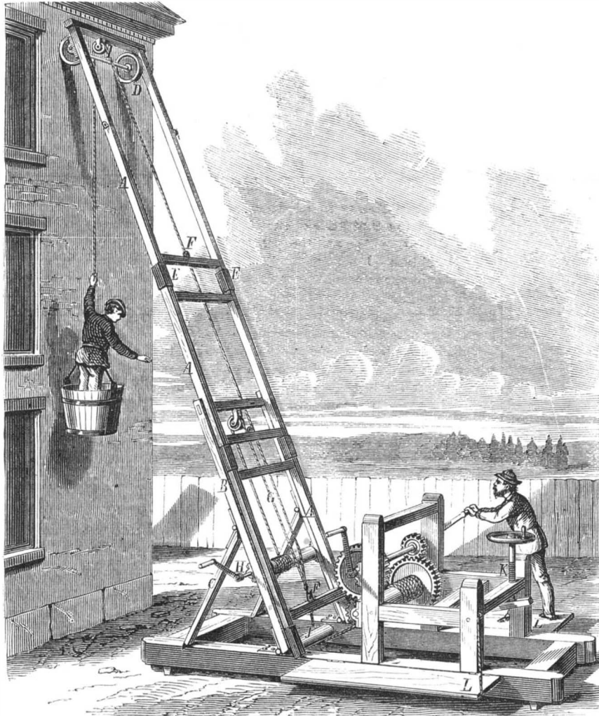
PATRICK'S FIREMAN'S AND BUILDER'S ELEVATOR.
