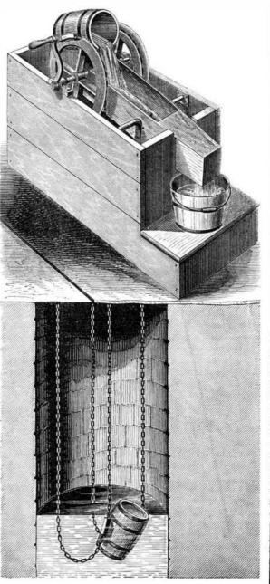
Our engraving gives an excellent idea of the device. Two grooved pulleys keyed to a shaft carry each an endless chain to which buckets are attached in the manner shown.
