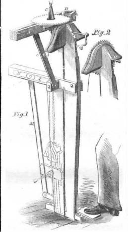
of the saw exactly over the angle in the anvil. For setting straight saws the ends of the teeth are placed against the brass guides, d, which open at a greater or less angle, and thus permit the tooth to project a greater or less distance past the angle in the anvil.
