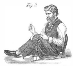
which the leg rest is adjusted. The weight of the leg is sustained by a spiral spring encircling the upright of the leg rest. The bar to which the supporting device is attached may be contracted or extended by means of a slot in the bar and a screw attached to the chair seat.
