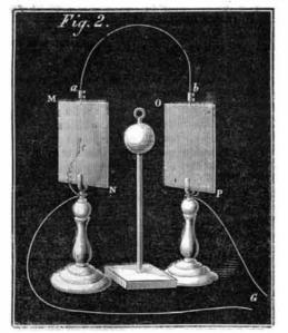
which will inform me which of these plates is heated. Suppose I heat this plate. Observe what occurs at the magnetic needle. I simply warm that plate by putting my finger upon it. The red end of the needle moves towards me. I cannot explain the wonderful power which moves the needle. It is what we call an electric current, and is produced by the union
