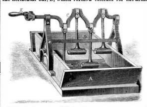
and, in combination with the cranks, gives the shoes a curvilinear motion, by which the dough is carried under them through the box in a direction corresponding with the direction in which the shaft is turned by the handle, E.
