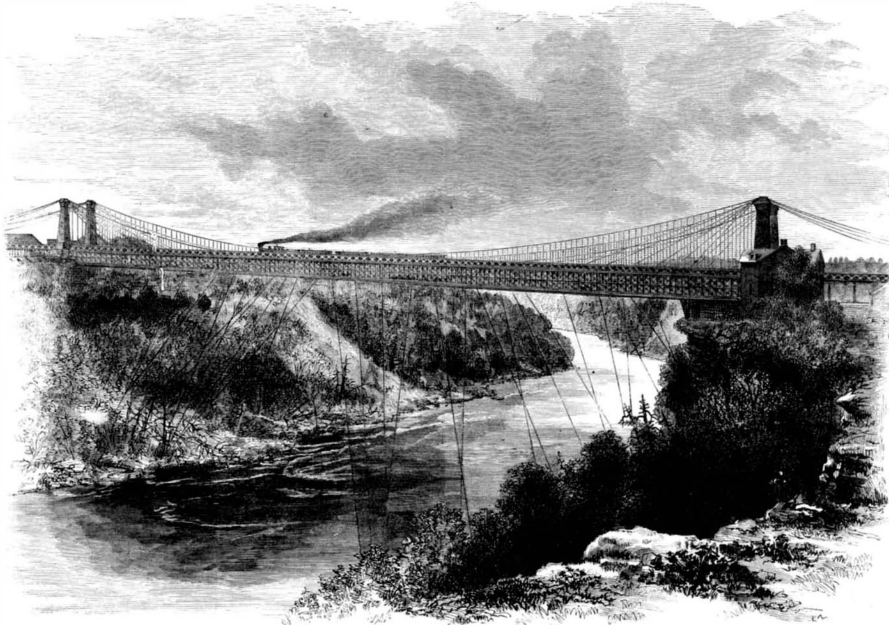
THE SUSPENSION BRIDGE ACROSS THE NIAGARA.
