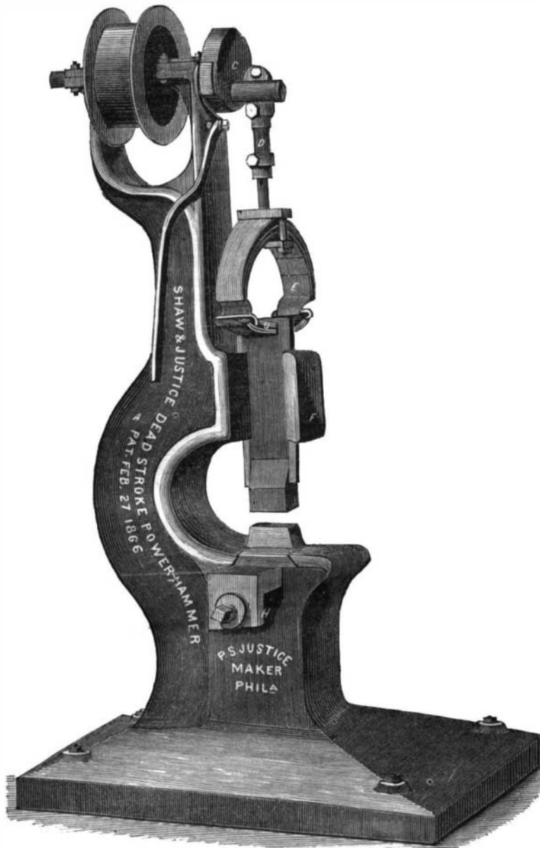
SHAW'S DEAD-STROKE POWER HAMMER.
