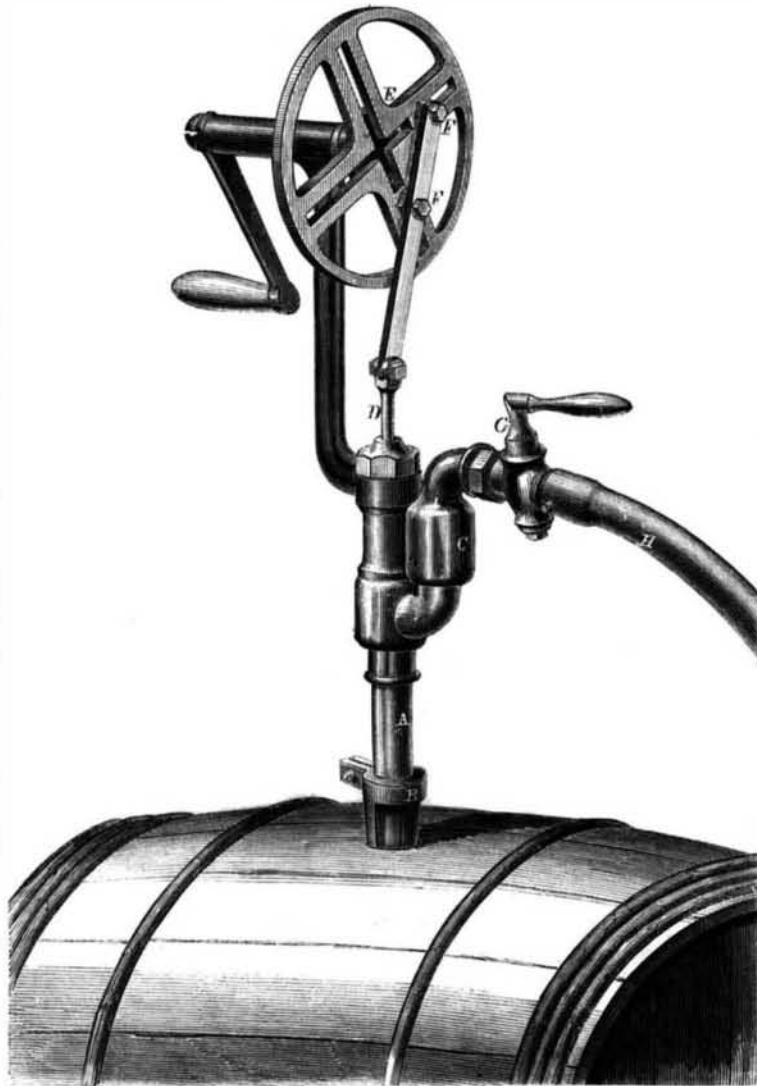
TULLY & REECE'S LIQUOR AND TRANSFER PUMP.
