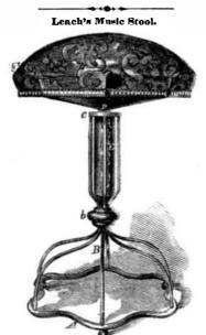
who is about to sit down. The screw, D, when between the rods. B. is covered with an ornamented case, E, so that the appearance of the stool is always graceful, tasty and convenient. They can be made much cheaper than wooden ones, and are in every respect preferable, as being capable of enduring infinitely more wear, and present an elegant piece of furniture as an accompaniment to a musical instrument.
