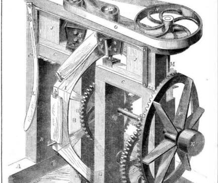
The want of a simple, cheap, and efficient | L, and toggles, secured to the slides, the hanstave-jointer has long been felt, especially for | dle being secured in any position by a rack, flour barrels, where a perfect joint is of great importance, as it not only protects the contents from injury, but adds to the strength | band wheel, N, the band, O, of which, passes of the barrel.
