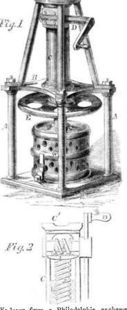
We learn from a Philadelphia exchange, that recently a man weighing 156 pounds, lifted, with the aid of one of these presses, t weight of 37,332 pounds, merely by ne gr the application of his strength to the lever 20 inches long, and the press weighed only 45 pounds.
