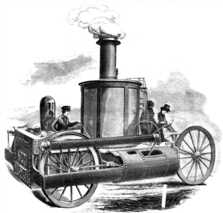
We present herewith a series of illustrations of the new self-propelling steam fireeugine, "J. C. CARY," built at the Novelty Iron Works, by Messrs. Lee & Larned, under a contract with the city of New York. This engine was brought out for its first public trial at the Bowling Green on the 5th inst., and again in the Park on Thanksgiving Day, the 18th inst., and its remarkable performance on both occasions has attracted to it an unusual degree of public attention.
