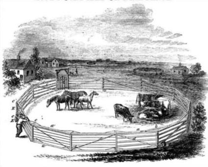
iron the rails, a', can be made of two boards, forming a T-shaped rail, or a square piece mortised into the posts, and connected together by the braces, b', which are held out from the posts by the blocks, e, that serve to make the connection more substantial than when the braces are straight. The brace, d,
