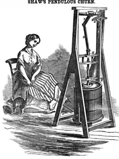
novel device for agitating cream, invented by back and forward motion, as in working a Charles A. Shaw, of Biddeford Me. and pat- pendulum, is far more agreeable, and is that ented December 9, 1856.
