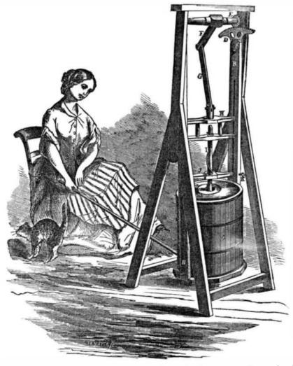
novel device for agitating cream, invented by back and forward motion, as in working a Charles A. Shaw, of Biddeford Me. and pat- pendulum, is far more agreeable, and is that ented December 9, 1856.
