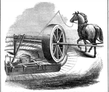
down, the drag then gathers the mortar | form us, that with the labor of one man and formed into a heap, if desired, or pushes it a horse, thirty casks of lime can be made down into the receptacle described, through into plastering or building mortar by it in a trap door in path A. The lime employed is previously slacked before it is put on the way, A. A few revolutions of the roller and drag mixes the materials.
