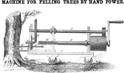
Power machinery for cutting down forest | wheel, L, which, in turn, receives its motion serious objection to the use in some otherwise the timber on a square league or more is disposed of.
