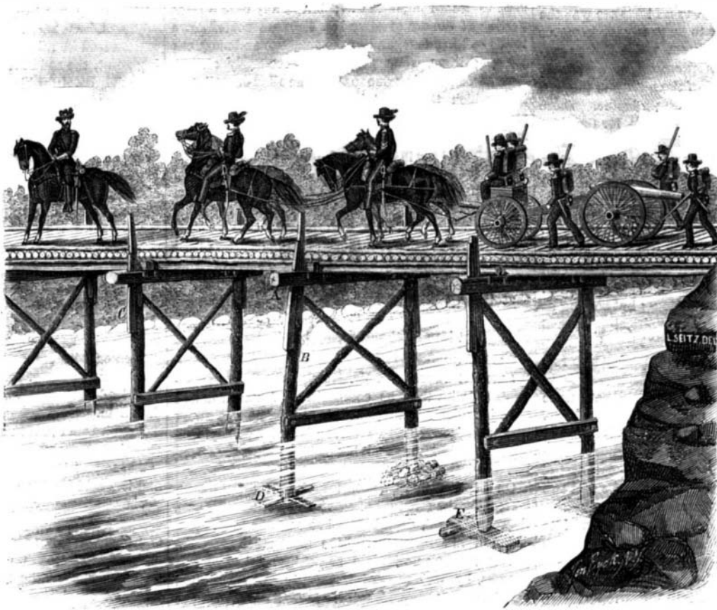
DERROM'S SYSTEM FOR TRESTLE BRIDGES.
