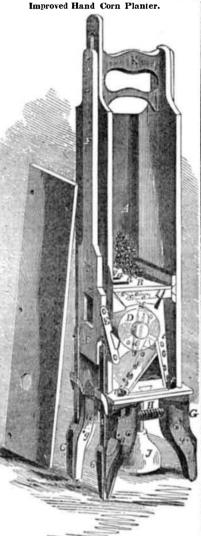
By S.L. Denny, Penningtonville, Chester Co, | at g. The lower ends of the movable legs are table, and the operator places his hand upon Pa.-This invention belongs to that class of kept closed against the ends of the fixed legs, planting contrivances which are carried in the in order to prevent the entrance of dust, by arrow 1, causing it to lean, as shown in the hand of he operator, the seed being planted means of spiral springs, H.
