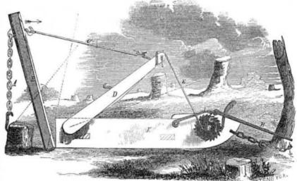
and prevents the ratchet wheel from turning | back. By the winding of strap E on shaft F, the lever, D, is brought down, strut, B, stump pulled. Most of the parts are attached to the sled, K, on which they are conveniently transported from place to place.
