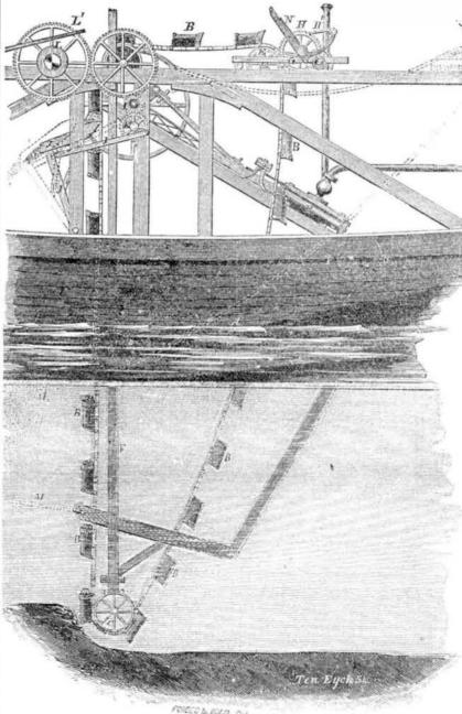
ets come in contact with any unyielding ob- steams off to the proper place; the traps are struction, the ways are allowed to rise, and the then opened and the load falls out. The in buckets pass over it without damage to the machinery.
